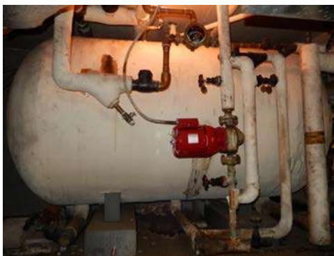
Indirect DHW Tank
