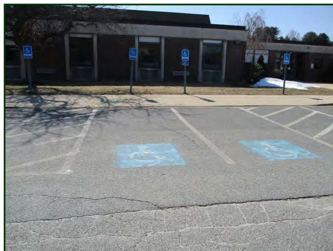
Photo #34: Accessible parking spaces, with faded painted lines & symbols, adjacent to the main building entrance. Note some asphalt pavement cracking
