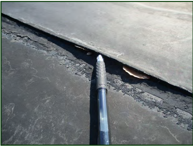
Photo #46: Aged roof membrane with deteriorated joint sealant & open joints to the weather
