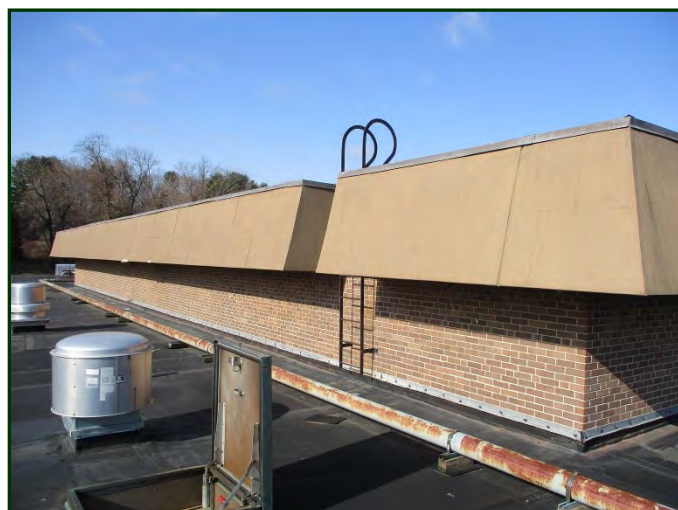
Photo #42: Raised portion at high roof with cracked stucco and brick veneer
