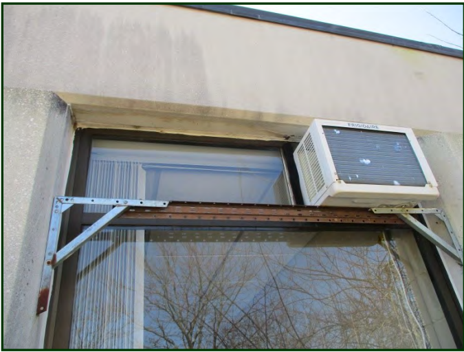
Photo #8: Through-window mounted air conditioning unit
