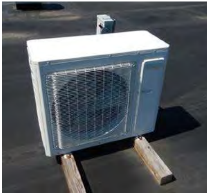
Superintendent's Office Heat Pump Condensing Unit
