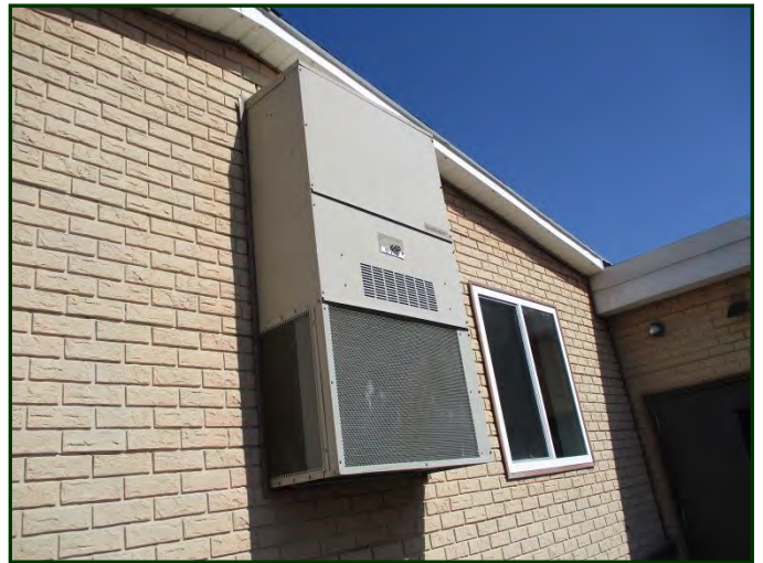
Photo #22: View of wall-mounted air handling unit & (faux brick) vinyl siding & vinyl-framed sliding windows
