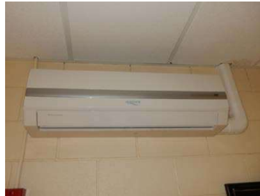
Superintendent's Office Heat Pump Evaporator Unit
