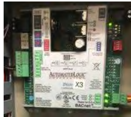
Typical ALC Controller for Misc. Exhaust Fans
