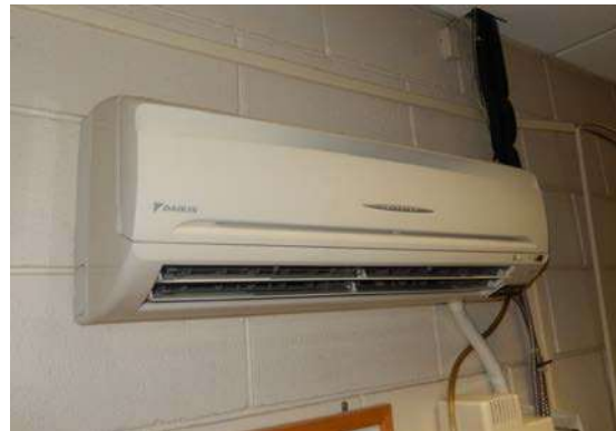
Server Room Evaporator Unit
