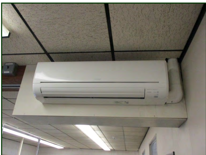
Photo #71: Ceiling-mounted ductless mini-split AHU in office area
