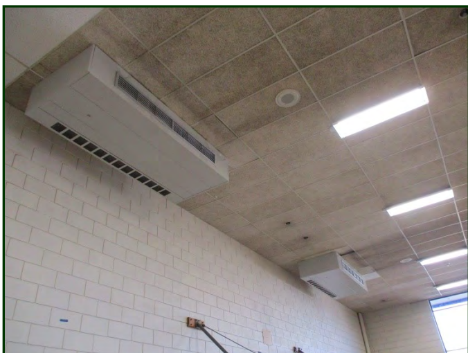
Photo #67: Ceiling-mounted air handling units in gymnasium with hot water coils. Note aged & stained ceiling tiles
