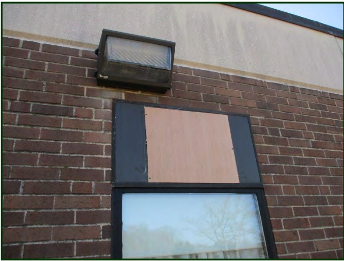
Photo #10: View of wall-mounted light fixture & blank off panel infilled with wood paneling (prior opening for AC unit)
