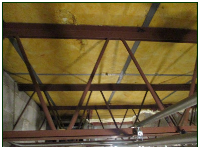
Photo #54: Superstructure with gypsum board roof decking on open web steel bar joist on load bearing CMU walls (predominately)
