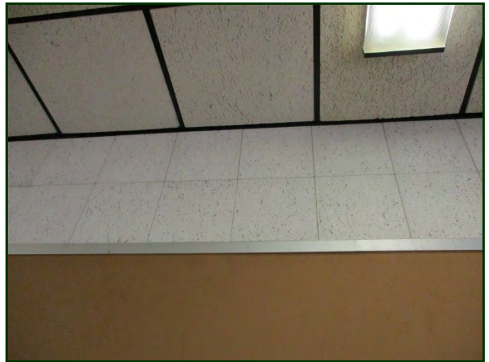
Photo #62: View of acoustical wall tiles in classrooms
