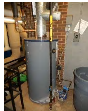
Natural Gas Fired DHW Heater
