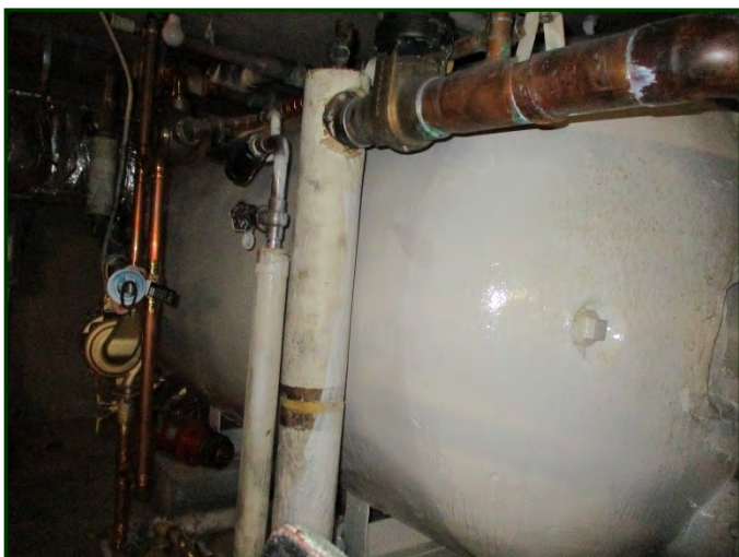
Photo #69: Original indirect-fired water storage tank used for heating months, in boiler room
