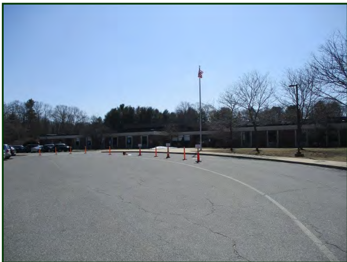
Photo #31: Asphalt paving at east side at drop off-pick up area with minor random cracking
