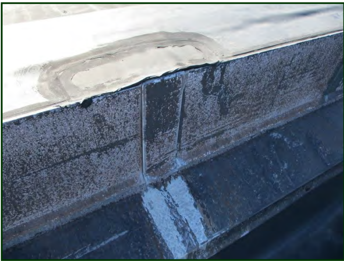
Photo #48: Metal plates at coping seams with open joints
