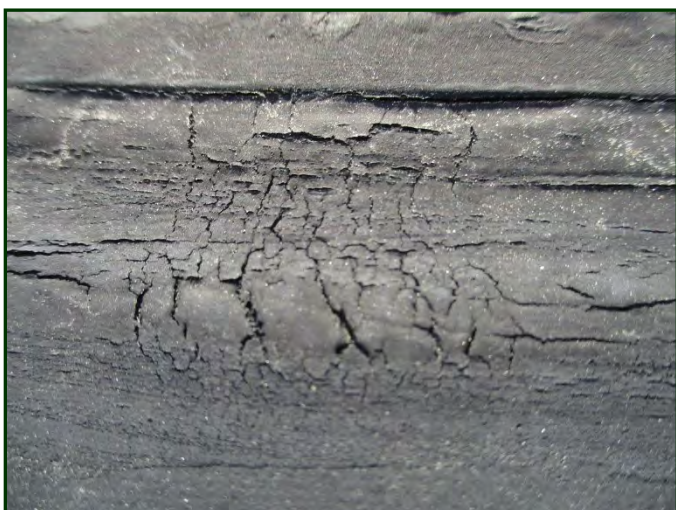
Photo #41: Aged and cracked sealant at historical patches
