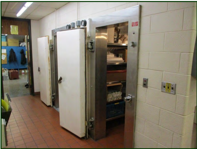
Photo #74: Walk-in cooler and walk-in freezer in kitchen area
