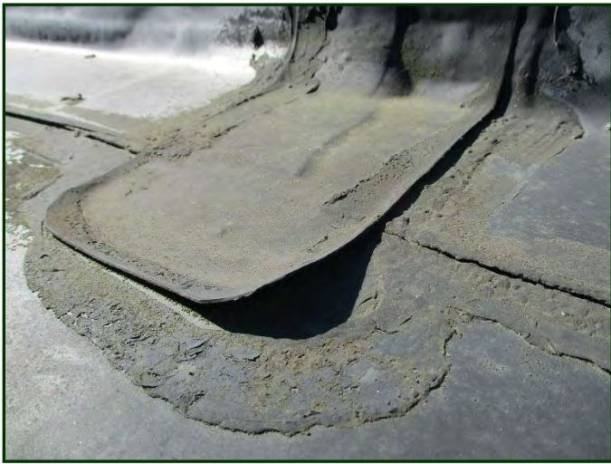
Photo #49: Historical patches lifting (with openings) at turned-up roof membrane
