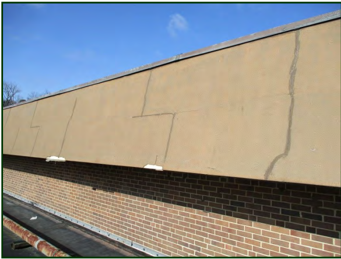
Photo #43: Close-up view of cracks in stucco at high roof
