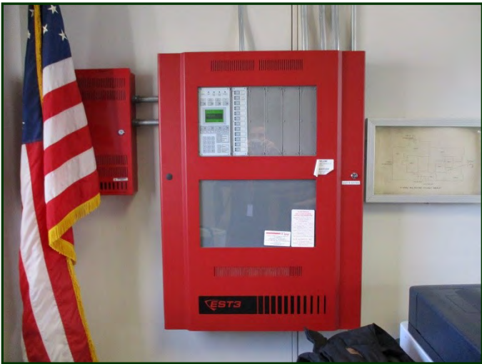
Photo #94: Fire alarm control panel in office adjacent to main building entrance
