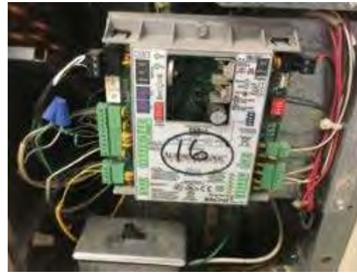
Typical Unit Ventilator Controller
