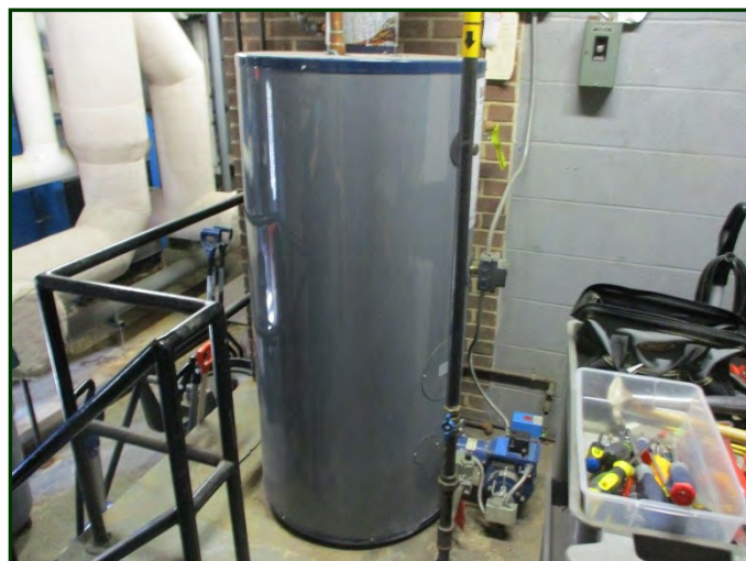
Photo #70: Gas-fired domestic water tank for non-heating months, in boiler room (circa 2016)
