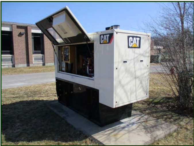
Photo #92: Diesel-fueled emergency generator on concrete pad at rear of building
