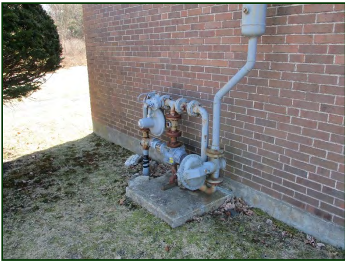
Photo #11: Natural gas service at southeast corner of building
