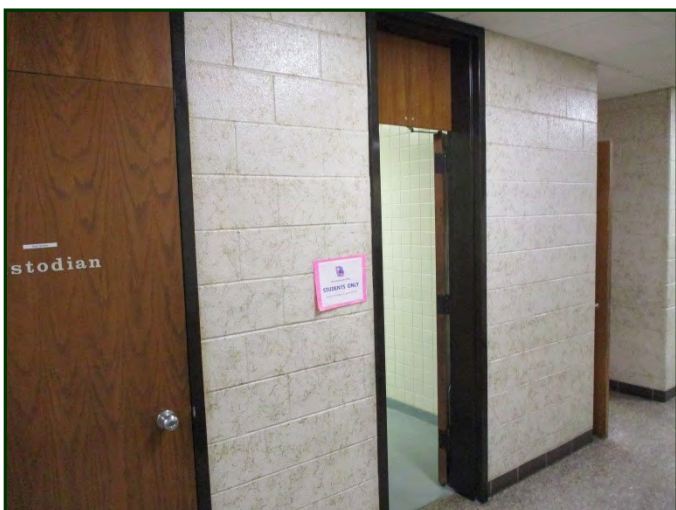
Photo #59: Student toilet room with non-accessible doorway (too narrow for ADA compliance)-typical
