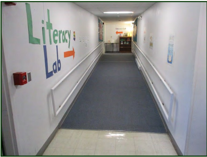
Photo #86: Ramp with carpet & metal handrails serving modular classrooms
