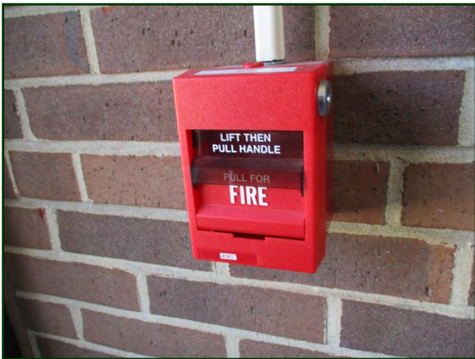
Photo #95: Manual pull fire alarm device
