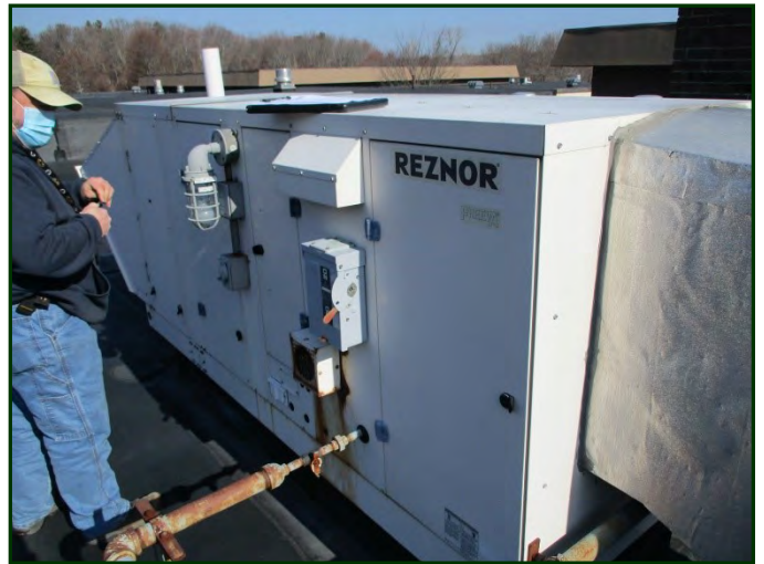
Photo #52: Gas-fired roof-mounted heater supplying tempered air to boiler room below (circa 2008)
