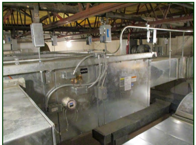
Photo #66: One of three air handling units on mezzanine (circa 2010) supplies heat & ventilation to library, hallway, auditorium & Learning Center
