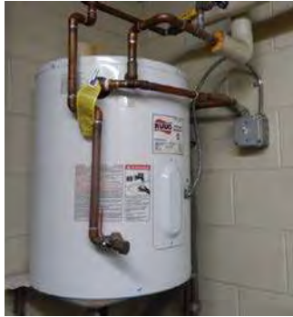
Electric DHW Heater
