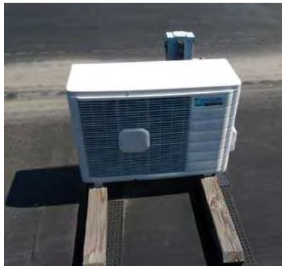
Server Room Condensing Unit
