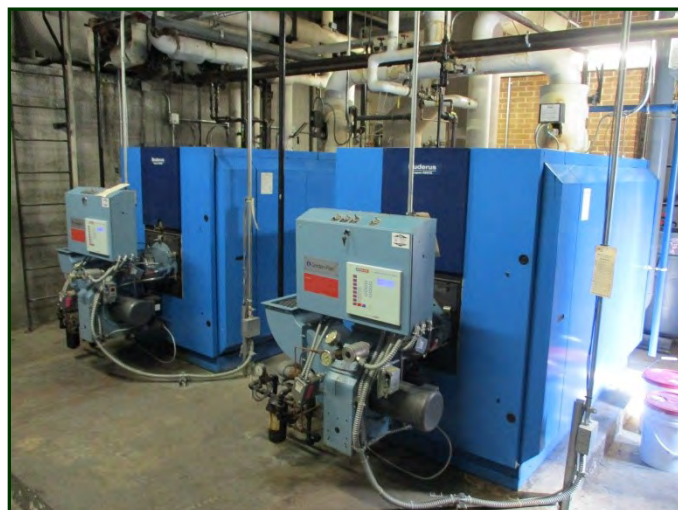
Photo #68: Gas-fired boilers in boiler room (circa 2006)
