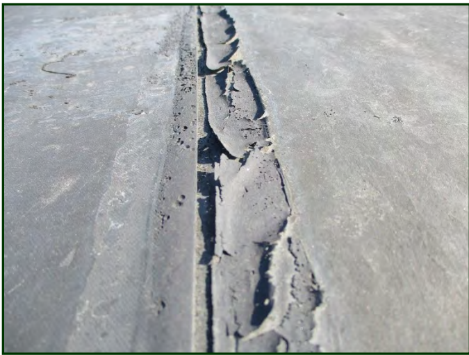
Photo #47: Close-up view of deteriorated joints in roof membrane
