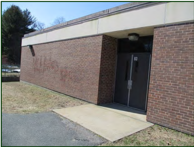
Photo #13: Egress doors at south elevation with soffit-mounted light fixture
