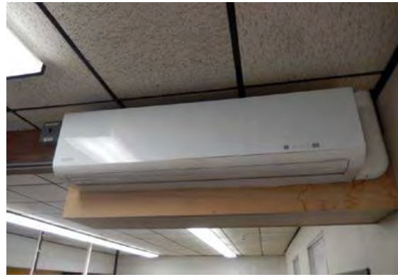
Superintendent's Office Evaporator Unit A
