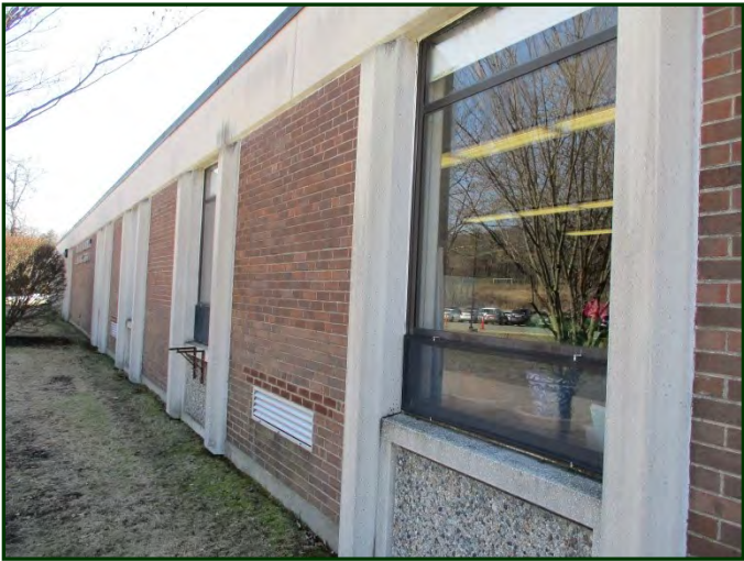
Photo #6: Close-up view of aluminum-framed windows, cast stone trim, brick veneer & thru-wall ventilation
