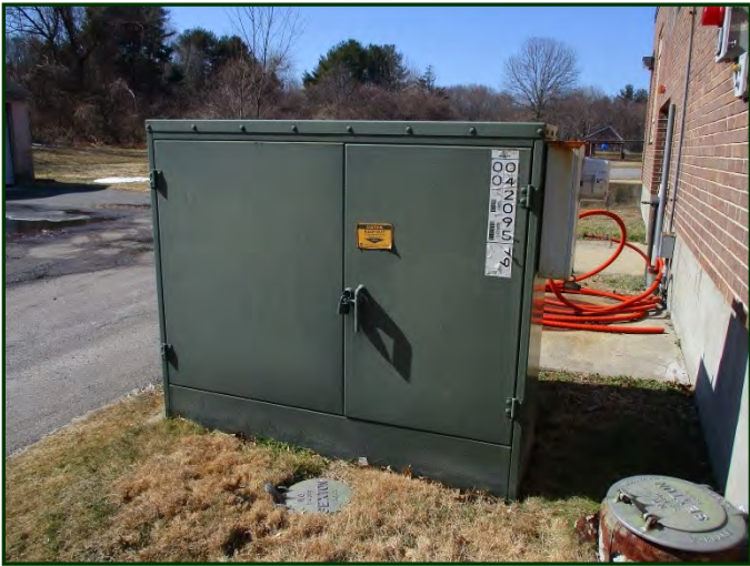
Photo #90: Pad-mounted electrical transformer
