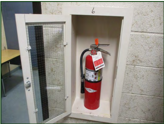
Photo #96: Fire extinguisher in wall cabinet with current inspection tag
