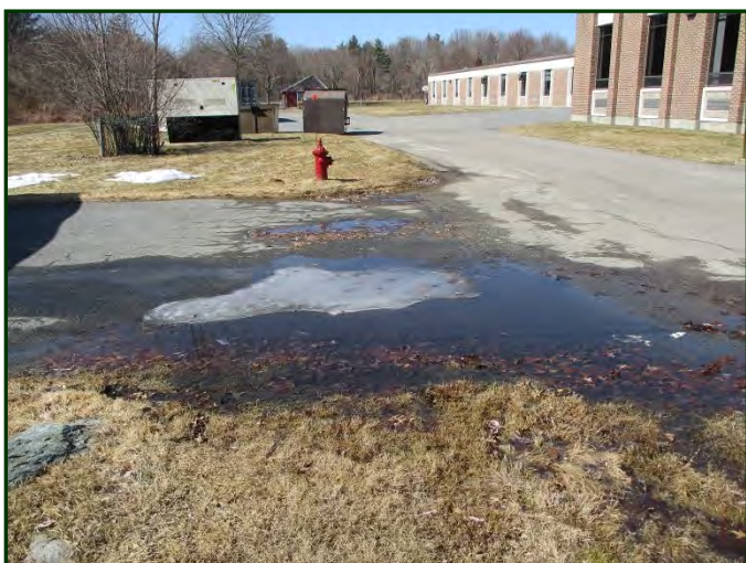
Photo #35: View of ponding water on asphalt pavement at west elevation
