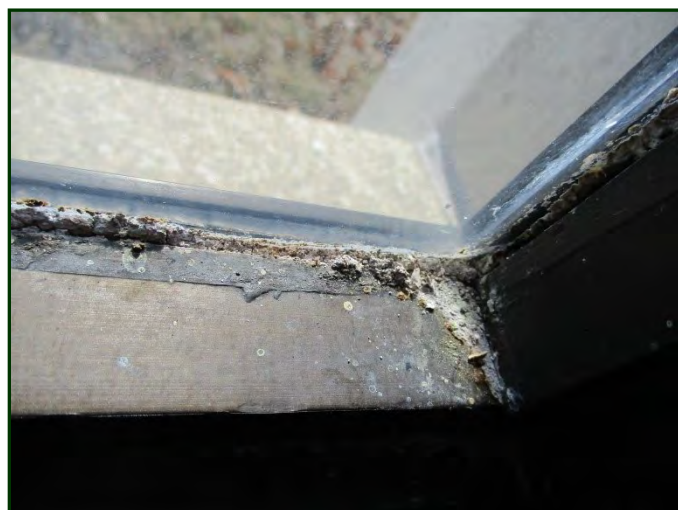
Photo #60: Interior view of aluminum-framed windows with deteriorated glazing (powdery & spalling) & aged gaskets
