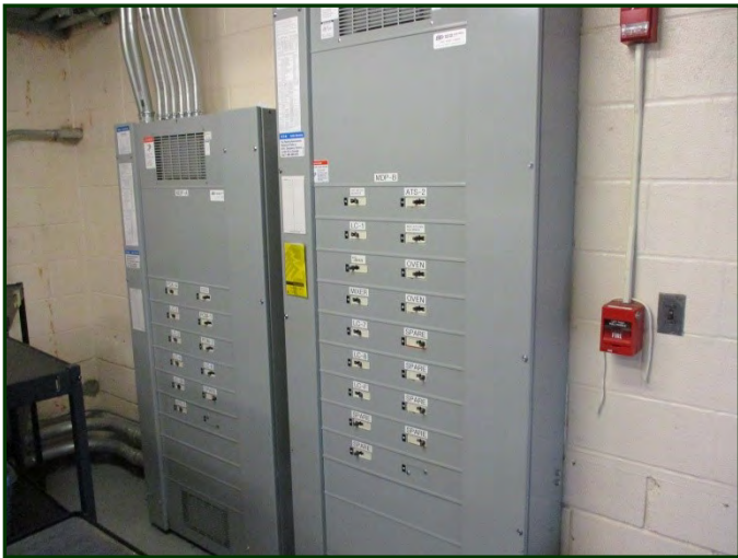
Photo #91: Main electrical switchgear
