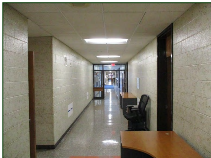
Photo #56: Corridor with (reported) VAT flooring, epoxy painted CMU walls and suspended acoustical ceiling system
