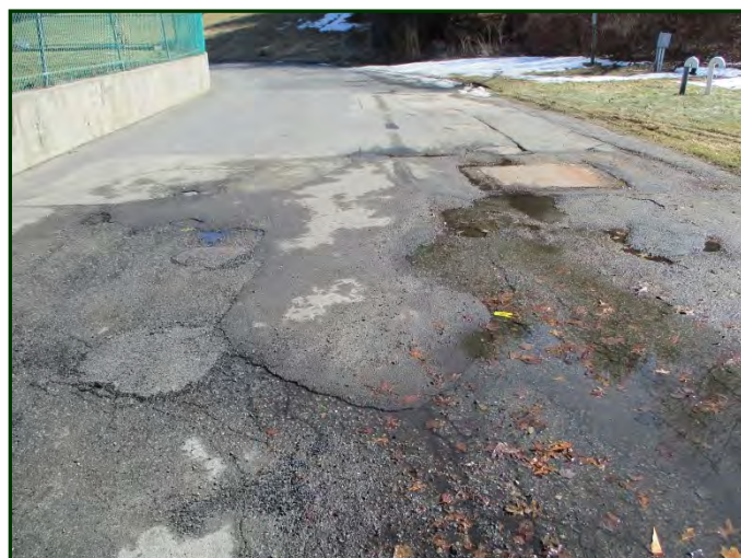
Photo #36: Continuation of ponding water at west elevation with some potholes, note septic system beyond
