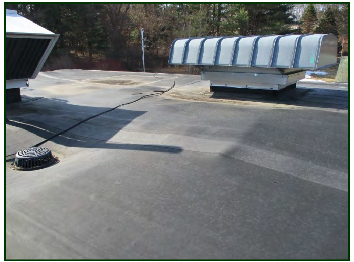
Photo #50: Severe tenting of roof membrane, preventing drainage to internal roof drains
