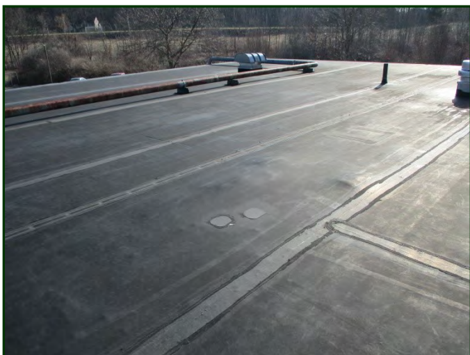
Photo #39: Overview of roof with an EPDM membrane (circa 1990). Note perimeter joints re-seamed & gas line beyond
