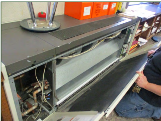
Photo #65: Newer unit ventilators (circa 2009 approximately) with hot water coils (supplies heat & fresh air) at classrooms-typical
