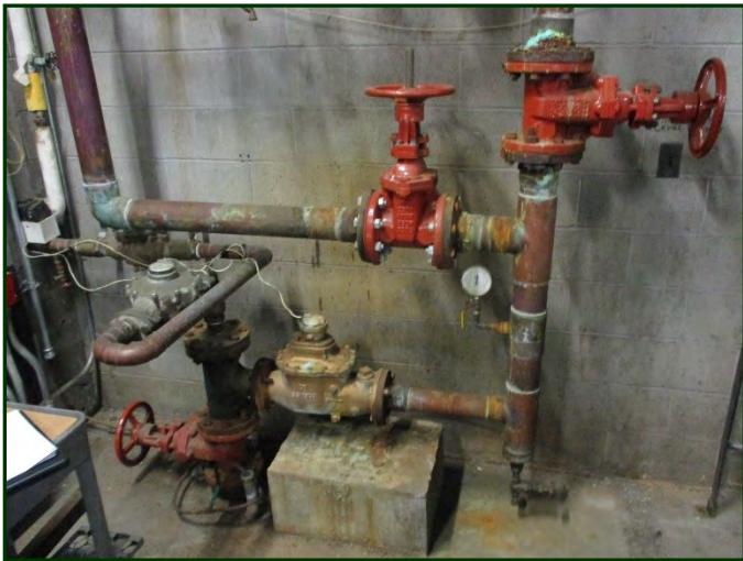
Photo #93: Domestic water service with backflow preventer in boiler room
