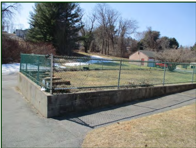
Photo #15: Raised area of lawn at the southwest corner with concrete retaining wall and chain link fencing
