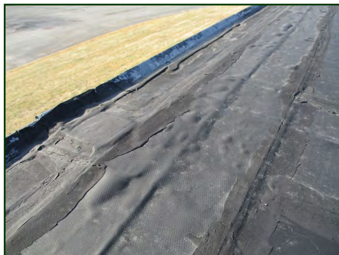
Photo #40: Edge of roof with aged and separating sealant at joints
