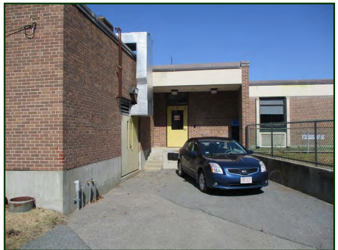
Photo #16: Concrete loading dock with bumpers at west elevation (rear of building). Note ductwork from roof to boiler room
