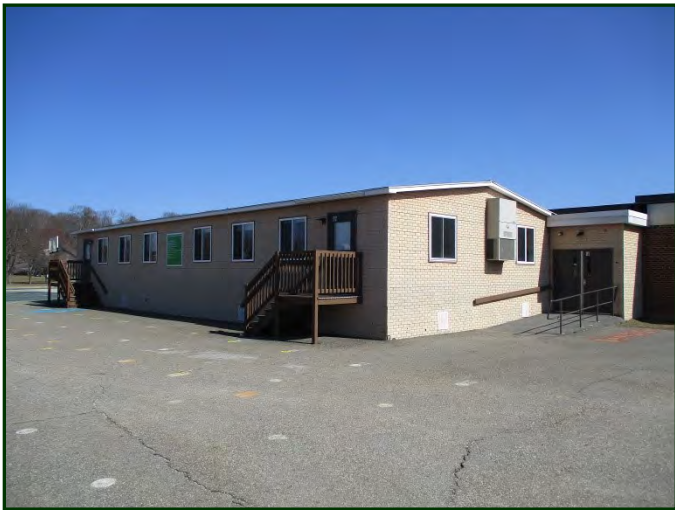
Photo #21: Modular classrooms. Note wood stairs & asphalt ramp with railings
