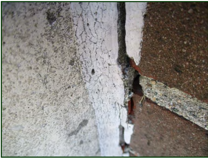
Photo #7: Close-up view of perimeter joint sealant at wall openings with aged, cracked and separating sealant
