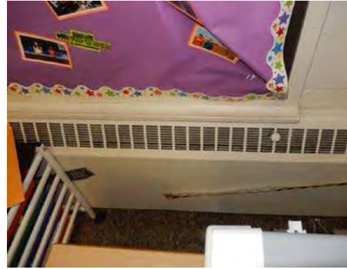
Fin Tube Radiation
