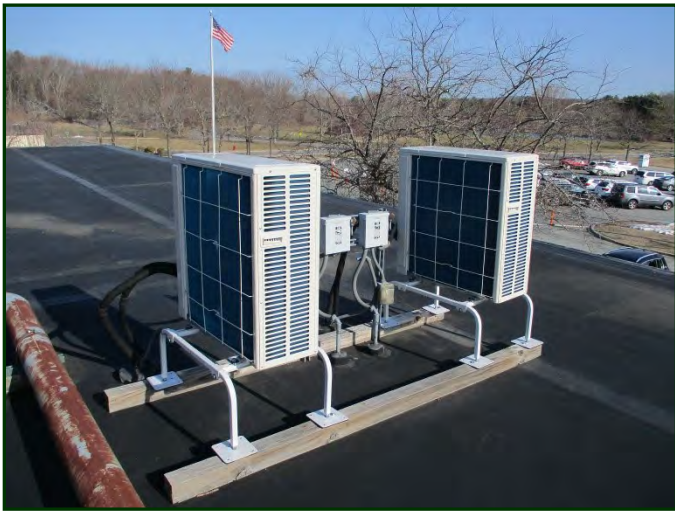
Photo #45: Roof-mounted condensers serving interior duct-less mini-splits (circa 2019)
