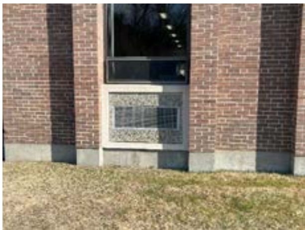
Typical Unit Ventilator w/ OA Louver
