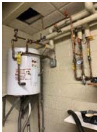
Electric Water Heater
