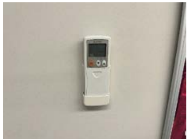
Split System Wireless Remote Thermostat
