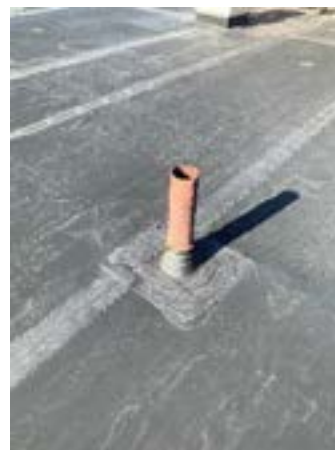
Vent Through Roof
