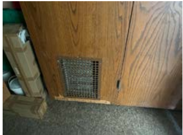
Typical Exhaust/Relief Grille
