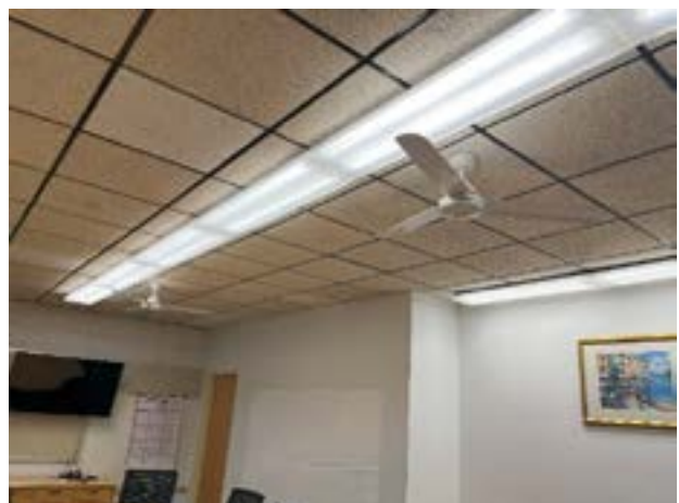
Ceiling Mounted Destratification Fans
