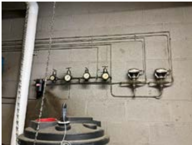
Abandoned Pneumatic Control System Gauges
