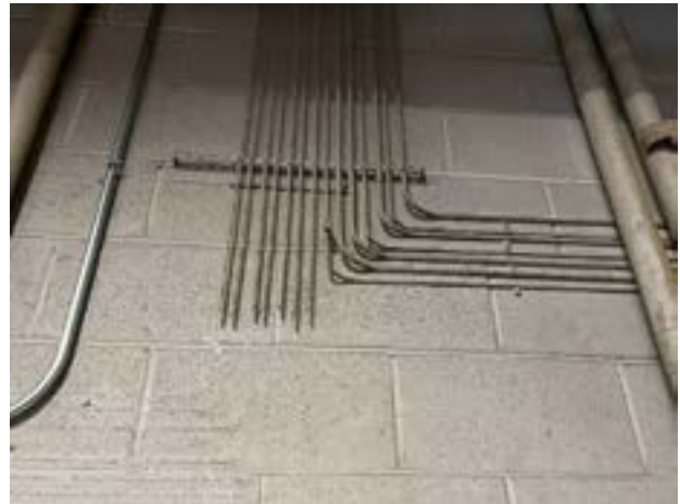
Abandoned/Cut Pneumatic Control Lines
