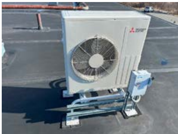
Typical Outdoor Terminal of Split Unit
