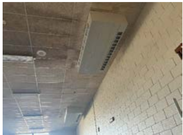
Typical Exhaust/Relief Grille
