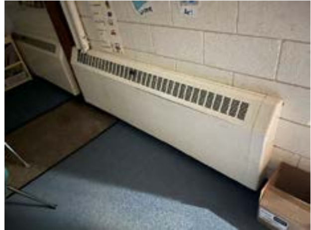
Typical Hot Water Fin Tube Radiation
