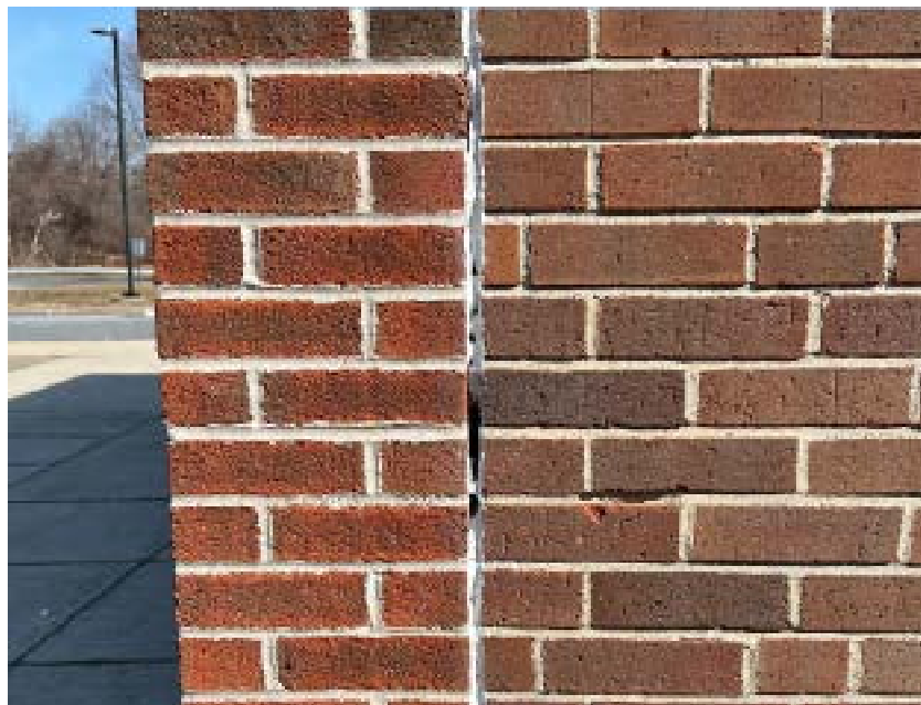
Figure 5 – Missing caulking at a Wall Joint
