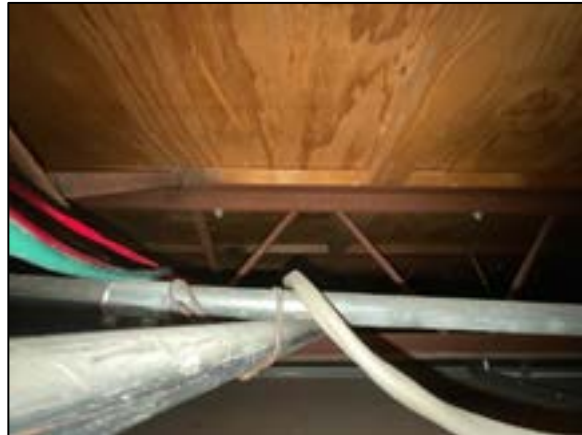
FIGURE 3: PLYWOOD ROOF AND STEEL STRUCTURE
