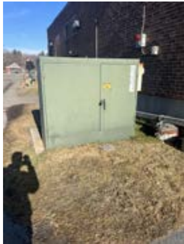
Pad Mounted Transformer
