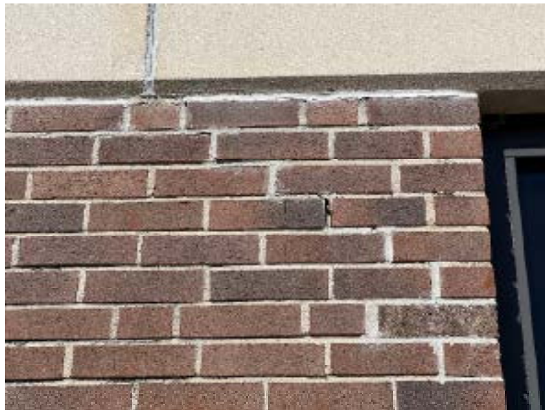
Figure 3 – Diagonal Crack Building on Brick Veneer
