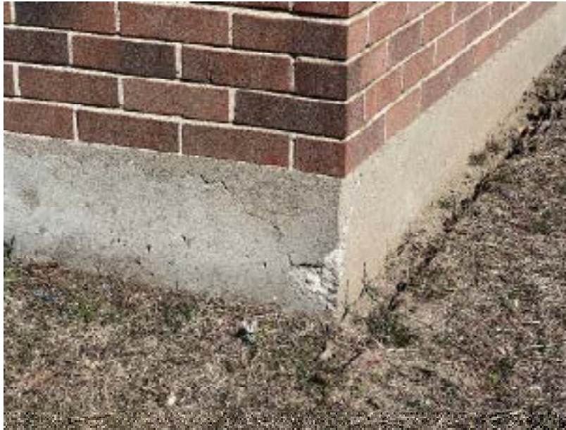
Figure 4 – Diagonal Crack in Foundation Wall Corner.
