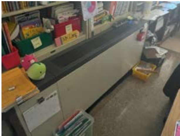
Typical Unit Ventilator w/ OA Louver
