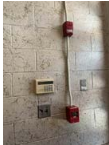
Pull Station/Horn Strobes
