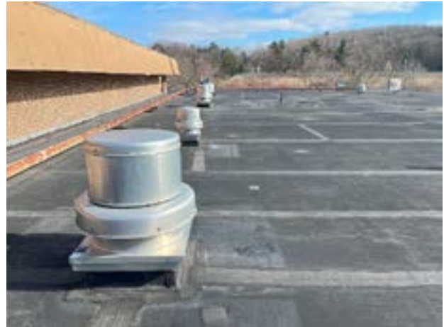
Roof Mounted Exhaust Fans
