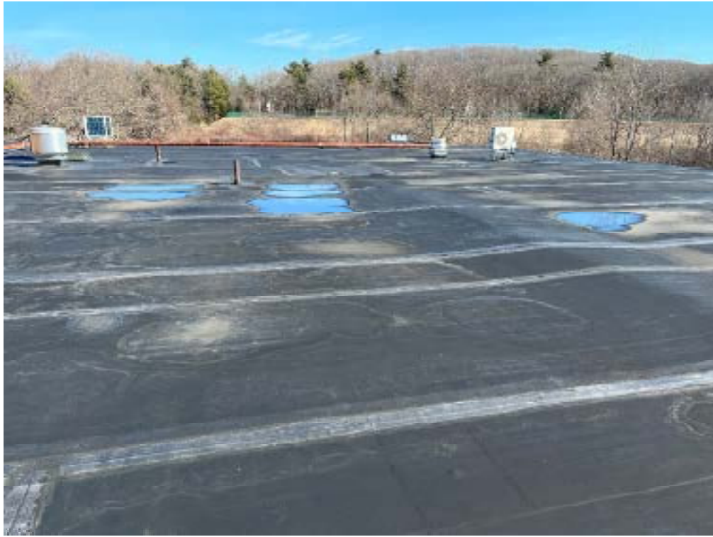
Figure 7 – Water Puddles on Roof
