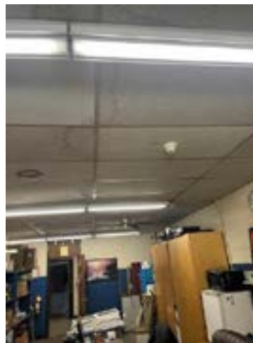
Fixtures Missing Lens
