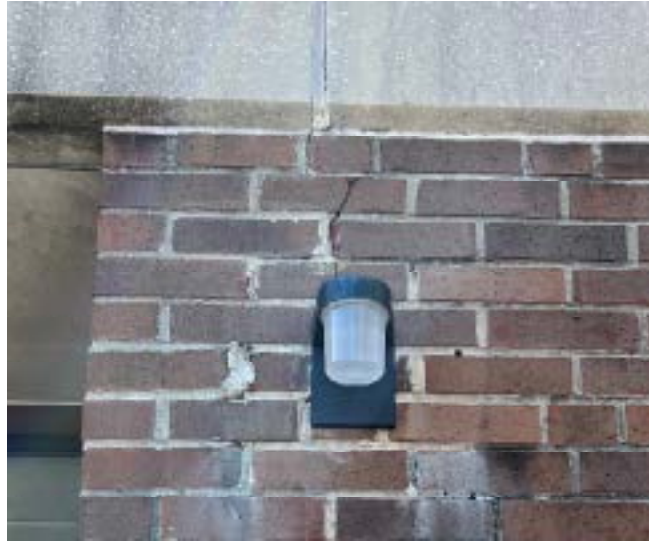
Figure 2 – Crack in Brick Veneer
