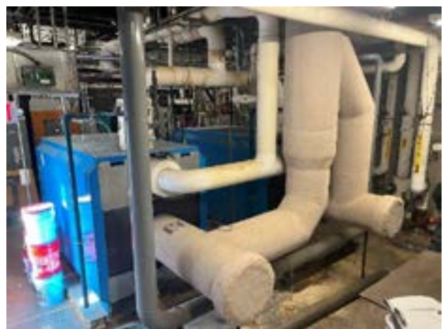
Insulated Boiler Venting to Chimney
