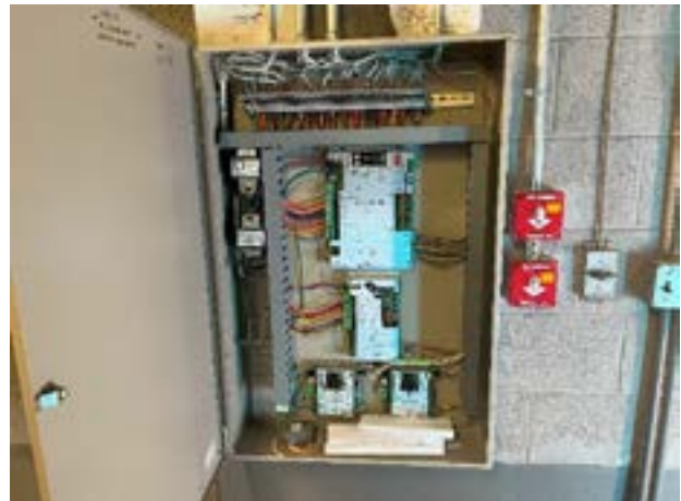
Controllers within Control Cabinet
