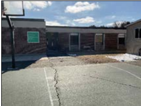
FIGURE 2: MASONRY EXTERIOR WALLS
