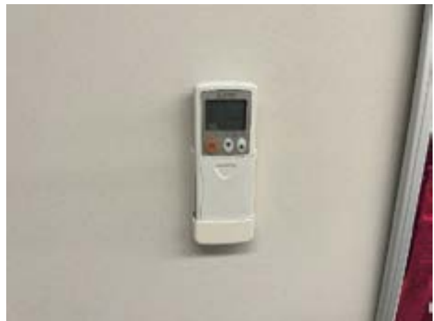
Split System Wireless Remote Thermostat
