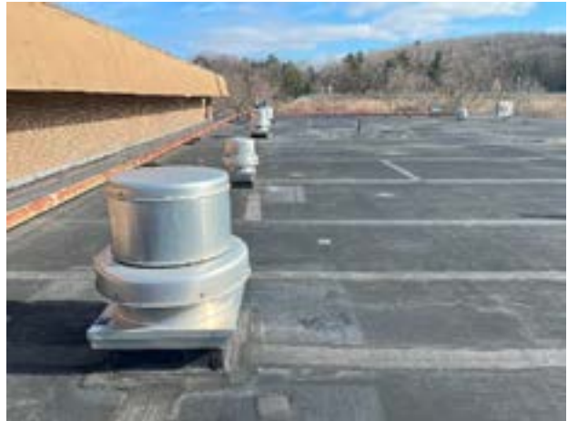
Roof Mounted Exhaust Fans
