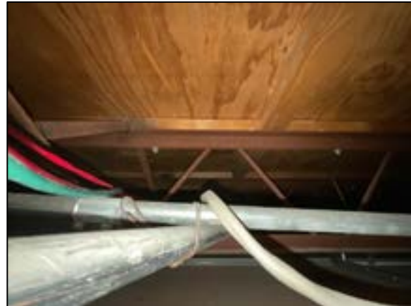
FIGURE 3: PLYWOOD ROOF AND STEEL STRUCTURE
