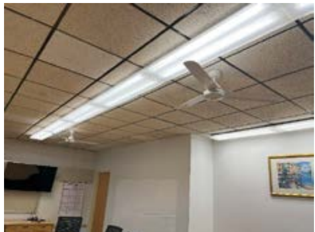
Ceiling Mounted Destratification Fans
