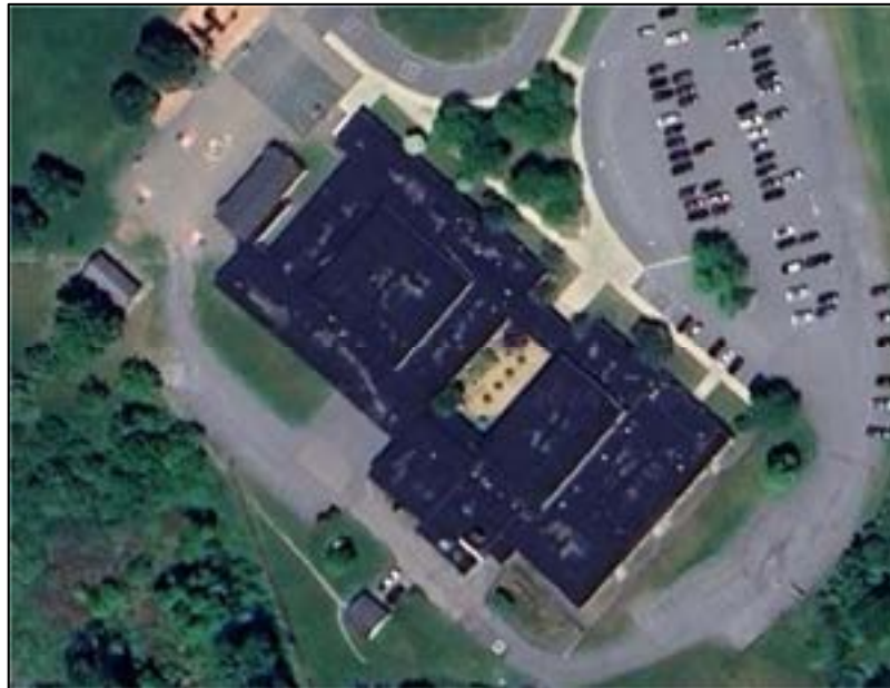
FIGURE 1: BUILDING SITE OVERVIEW
