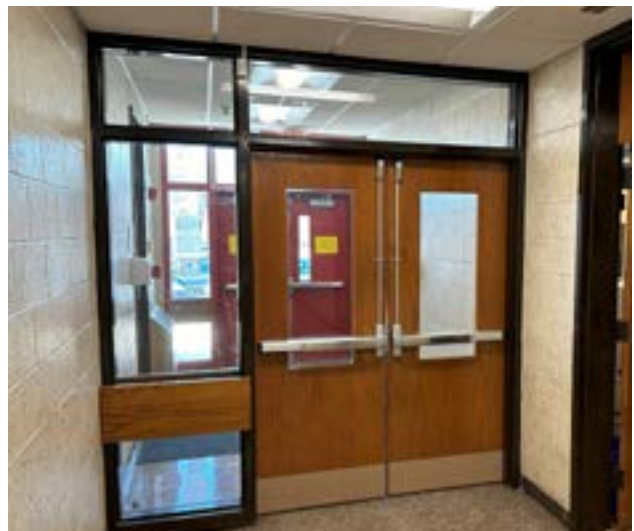
INTERIOR VESTIBULE DOORS
