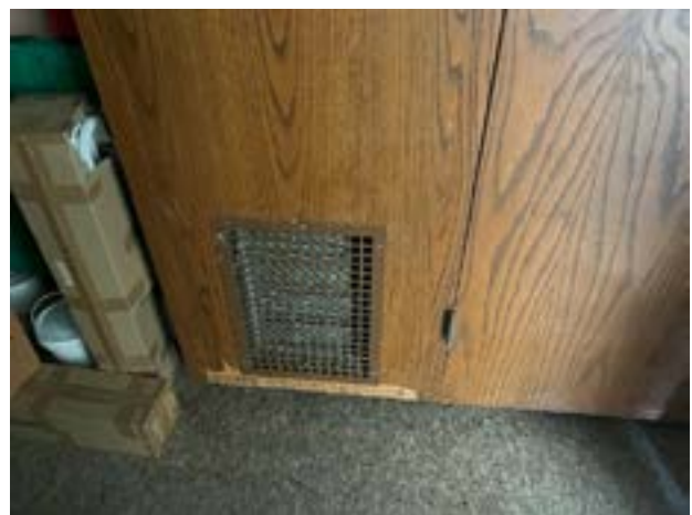
Typical Exhaust/Relief Grille
