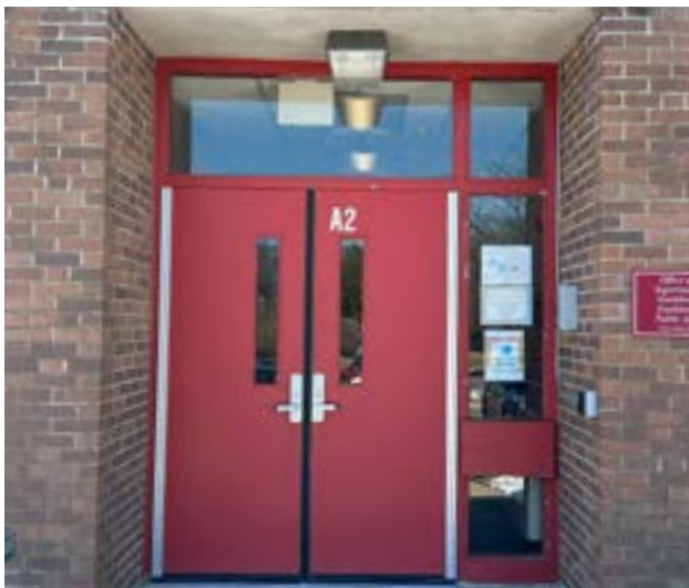
EXTERIOR ENTRANCE DOOR
