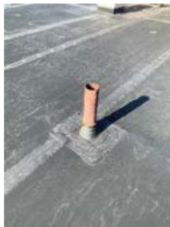
Vent Through Roof
