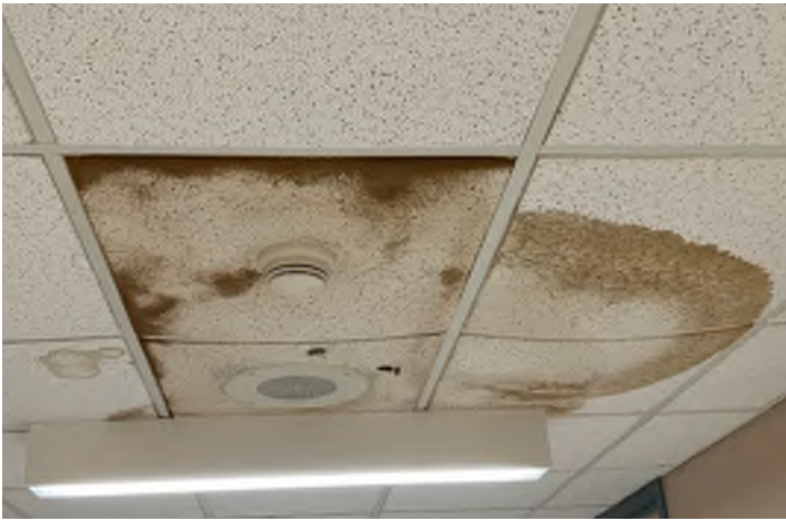
Ceiling damaged by roof leak
